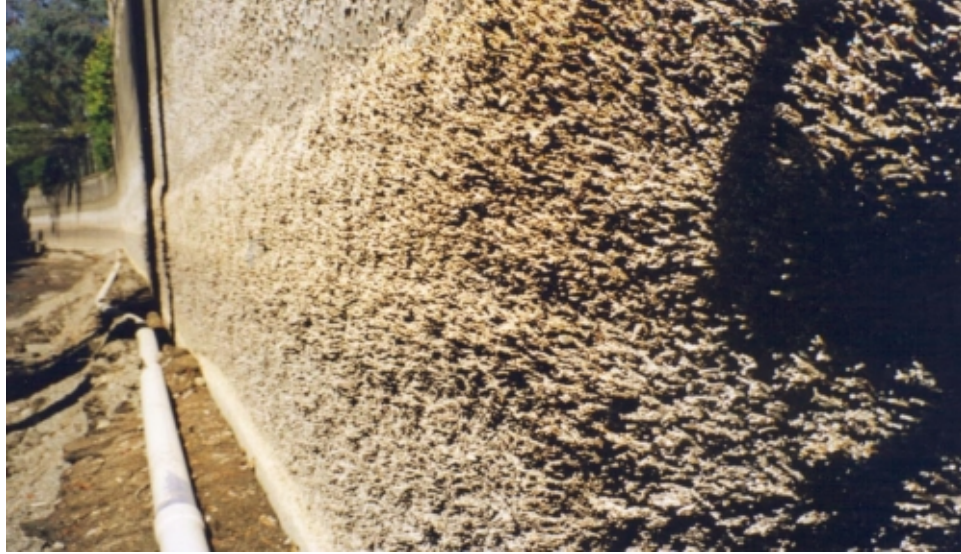
Figure 4. Tube worm and barnacle growth Station 323+00
